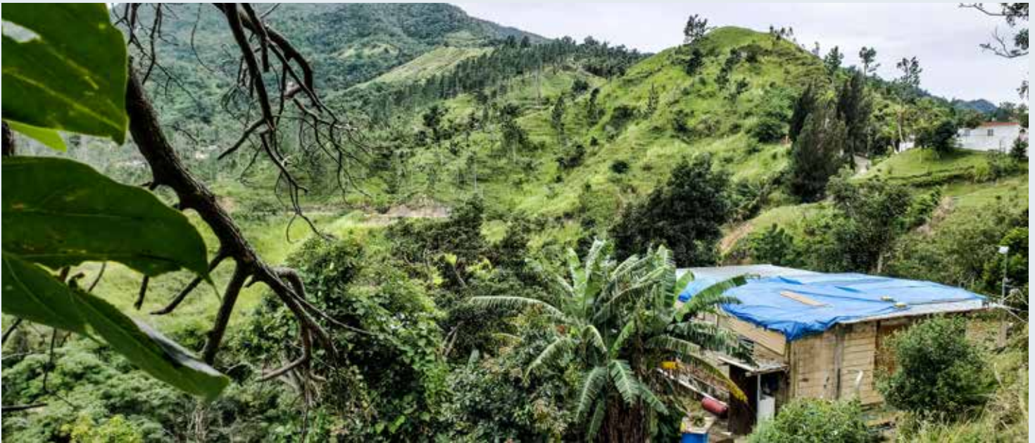
In remote villages like Jayuya, Puerto Rico, many house still needs to be repaired. The blue plastics roof where provided by FEMA in most cases, but also by NGOs. Photo: Fernando Briones.
