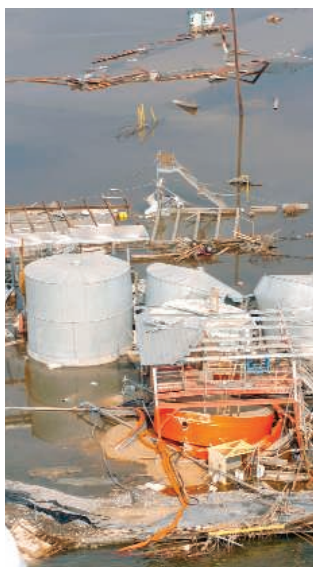
Damage to oil storage tanks in Cameron, Louisiana, caused by Hurricane Rita.
