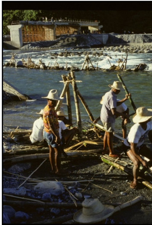
Figure 3. Zanjera San Marcelino farmers re-building bamboo, stone and brush dam (INIP Madongan Dam under construction in background). Source: Photo taken by Ruth Yabes, 1985.
