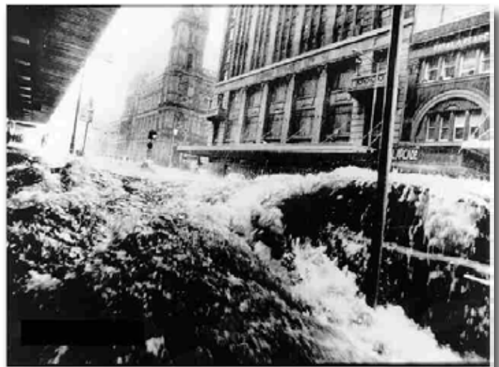
1972 Melbourne flood – Elizabeth Street. Photo courtesy of the Commonwealth of Australia 2009, Bureau of Meteorology (ABN 92 637 533 532).
