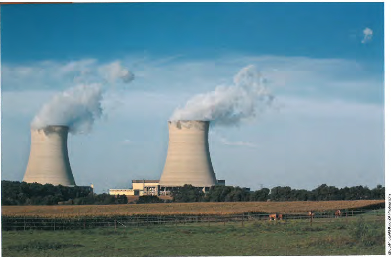
Cooling towers from the Byron, IL, nuclear Power Plant.
