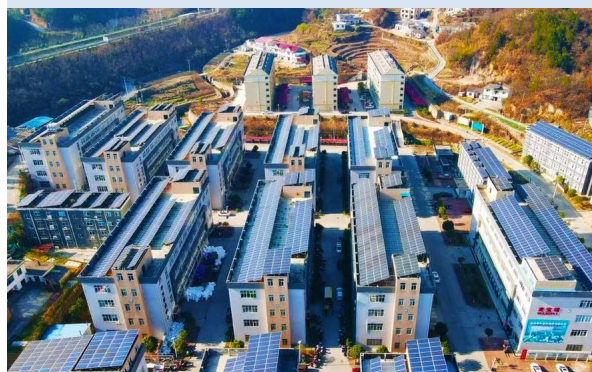
China added around 40% of the world's new solar panels last year, with large numbers of rooftop installations. Photo: Getty Images.
