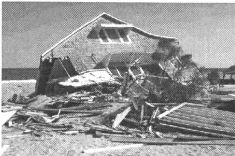
Some beachfront property became uninhabitable due to damage from Hurricane Fran in 1996. (Photo courtesy of FEMA.)
